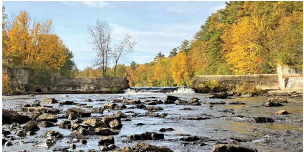
Looking upstream at the Indian Rapids Dam on the Saranac River during the fall of 2023
