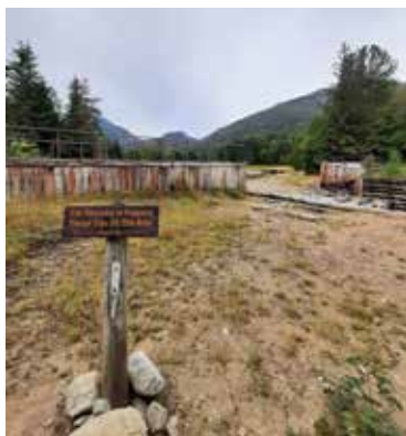
Remnants of Marcy Dam, High Peaks Wilderness Area, destroyed by Hurricane Irene
