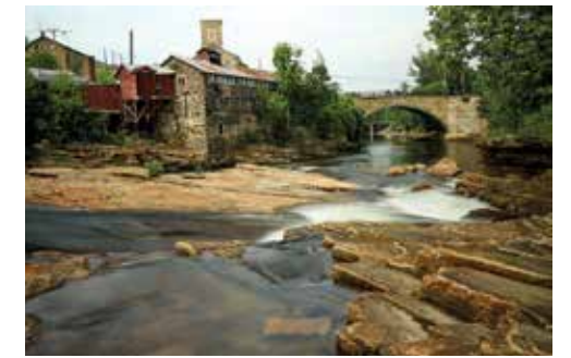
Anderson Falls and historic stone arch bridge in Keeseville, Town of Chesterfield
