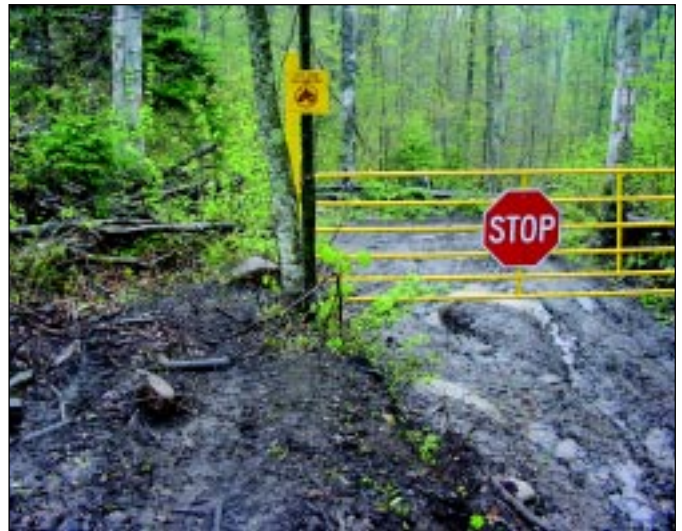
This barrier was erected in the Aldrich Pond Wild Forest to prevent all-terrain vehicle traffic from entering sensitive areas from legal trails. Last summer, it was pulled down by ATV-riding vandals.
